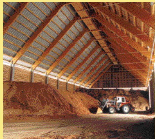
Fig. 3: Wood chips storage facility for biomass district heating plant, Bad Mitterndorf/Austria (Courtesy of LEV, Austria)
