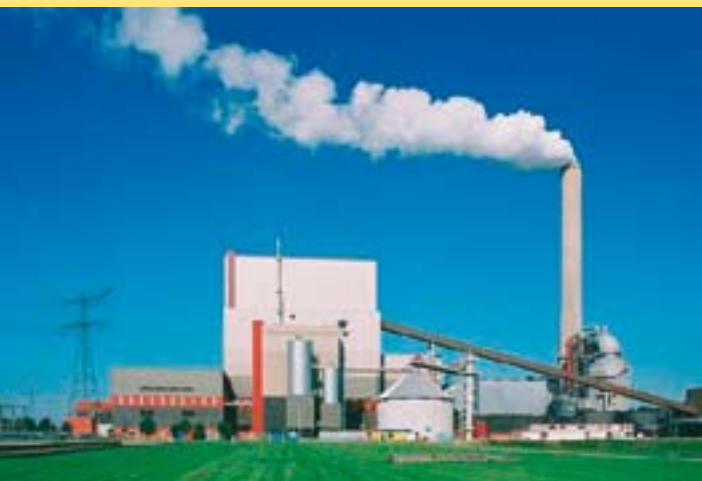
The Amer biomass co-firing power plant in the Netherlands. Courtesy Essent, the Netherlands
