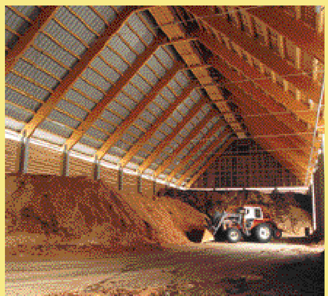
Fig. 3: Wood chips storage facility for biomass district heating plant, Bad Mitterndorf/Austria (Courtesy of LEV, Austria)
